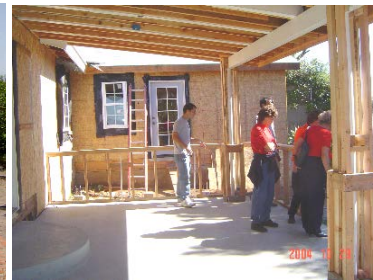
Remodeled back porch
